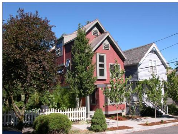
The City of Portland recently completed a design contest for more compatible skinny homes. This home was built using one of the winning designs. Advocating for improved design standards is one way we can ensure more compatible infill like this occurs in North Tabor.
